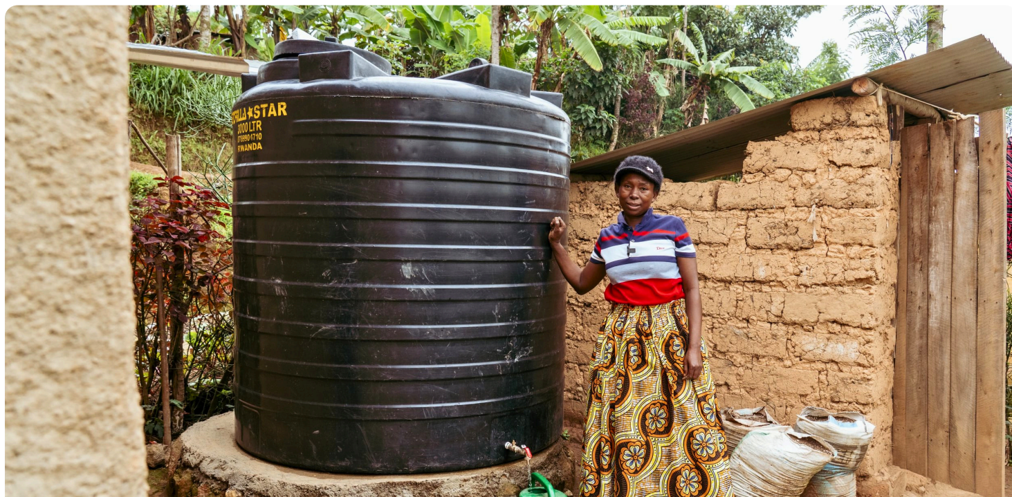
Alphonsine, a Kwigira project participant, with her new water tank that stores rain water
